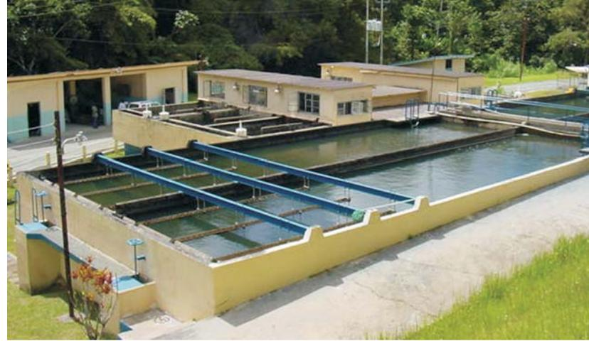
The final stage of the water treatment process is the addition of lime, to counteract the acidity of the water and the injection of chlorine to destroy any disease-causing bacteria.
